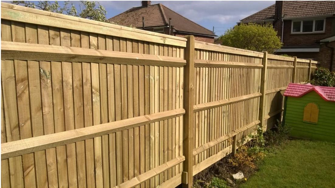
The next book will be on fences - eventually. I have to admit, I am having writers block. Not like me at all. But what do you think of this fence (image courtesy of Keighron Fencing in the UK). The rail is a split 75x75 which gives good water shedding and good thickness in the centre for fasteners. Does anyone know of this type of rail being used commercially in Australia. I expect my hardwood would not stay straight. Do you have any insights to share.
