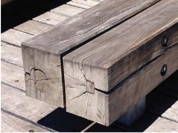
Firstly what is right with this design is that it is not bolted through the top allowing moisture into the heart. That can cause early degrade.
