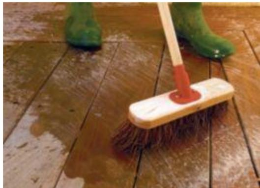
**Step 4.** Rinse off thoroughly with clean water using a hose or watering can, ensuring you've washed away all the residues. Allow time for your deck to dry out completely before you apply Tanacoat. Drying time will vary depending on weather conditions.
