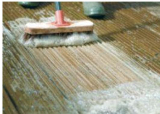
**Step 3.** Rinse off thoroughly with clean water using a hose, ensuring you've washed all residues away. Allow your deck to dry before you apply Tanacoat. Drying time will vary depending on weather conditions.
