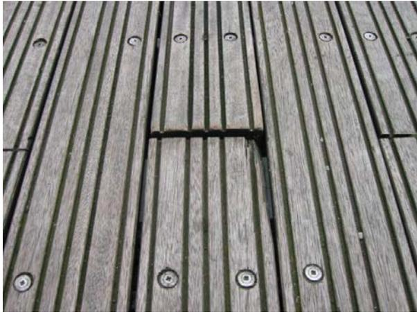
Building commercial decks with lineal decking and face fixings simply does not work if you want a trouble free deck that reaches its maximum possible life. The designer of this deck I saw in York UK recognised the problem and tried to sort it by overhanging about 220 mm and connecting the ends of the decking with wooden dowels. I would not say a complete success. Our Australian climate would quickly see decay where the dowel enters the end grain.
