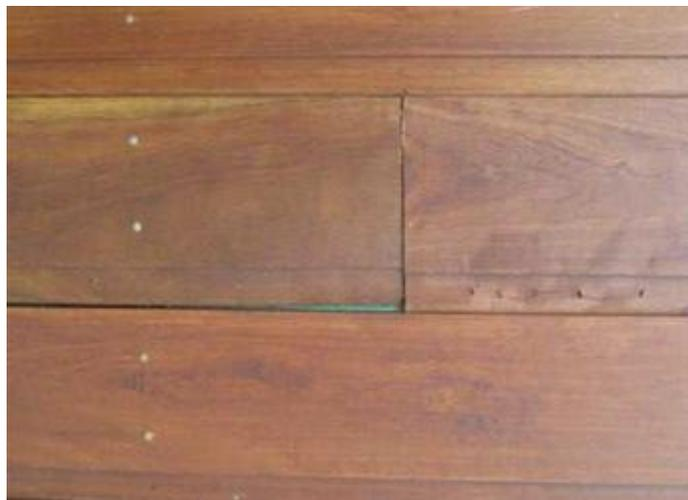
boards and produce dressed products from it and prepare yourself a claim. The image to the right shows recycled spotted gum which has shrunk so badly it that the shiplap is no longer lapping and you can see the insulation underneath.
