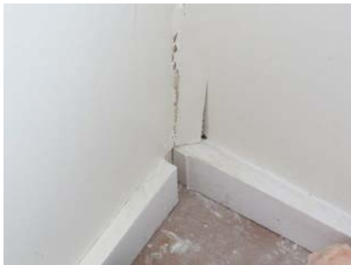
Damage to walls from expanding timber - Image courtesy of Colin Mackenzie
