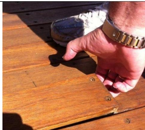
Broken screws in steel joists
