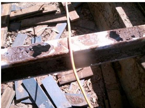
Badly rusted steel joist
