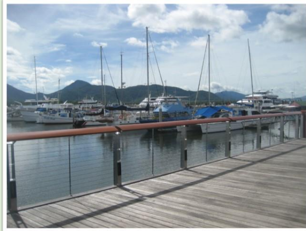
A very well designed handrail
