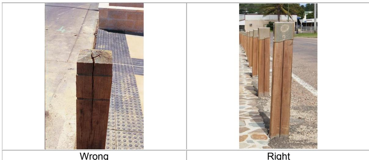
Sawn heart centre hardwood can have more issues than natural rounds. Because the outside is losing moisture and shrinking and the inside is still moist and so remaining
