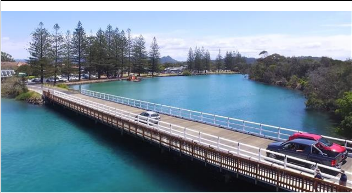
Restored South Arm bridge at Brunswick Heads
