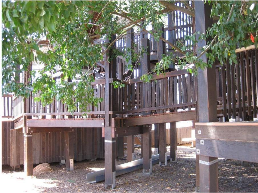
The decks generally follow the advice in this guide for best practice in construction with 120x35 mm decking laid on 75 mm joists with 14# screws installed in a staggered alignment. Posts are installed in stainless steel stirrups and all the fasteners are stainless. The playground is shown during construction in Figure 121 and note the use of conventional fasteners, not tamper resistant.
