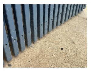
I saw this job recently. The battens on the left are fastened about 450 mm from the end and have moved badly. Those on the right-hand image are fastened about 150 mm from the end and are stable. Unsupported ends have a mind of their own and you need to consider this distance in your design. If I was designing a boardwalk without a kerb I would not have any more than 150 mm beyond the screw, if it had a kerb I would allow the length to extend to 200 mm as the movement will be hidden by the kerb.
