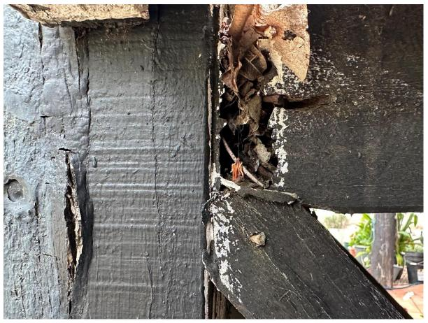
The lower durability of the timber when constantly wet means you should be very cautious of weather exposed housed joints. The image is from a set of steps made from kwila/merbau.
